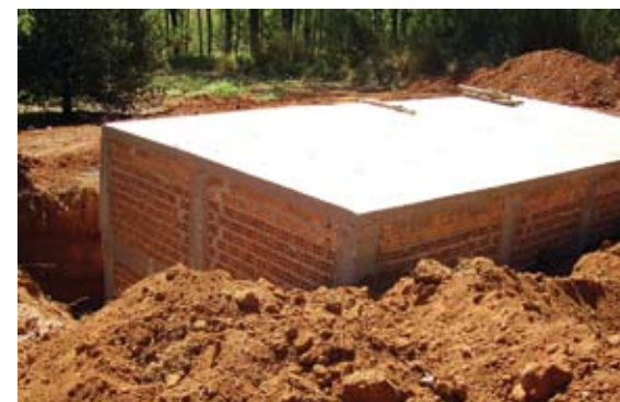
Construction of septic tank on certified property
