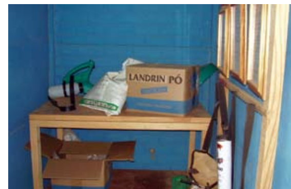
Worst situation of pesticide storage in certified companies (little space and boxes of anticide in direct contact with the floor).
